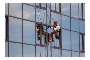
The rope access technician has none of these limitations. Ropes can be made to any length so that the tallest points of structures can be reached. Set up and tear down is so quick that a team of two can perform a hands-on evaluation of one façade of a 20-story high rise in one day. Conversely, if there is a need to have non-destructive testing performed at a singular location, that same team could be in and out in under an hour. The rental charge for a manlift alone would be costlier.
