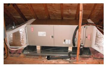
Figure 4 - Ducted split system - indoor air handling unit.
