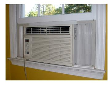
Figure 2 - Packaged window air conditioning unit.
