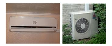
*Figure 3* - Split system indoor evaporator unit (left) and outdoor condensing unit (right).
