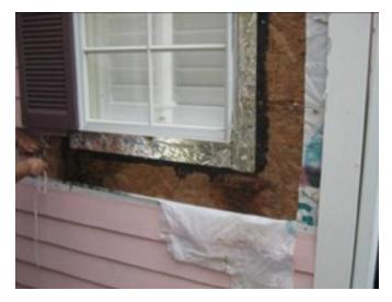
Figure 6 - Limited deconstruction below window
