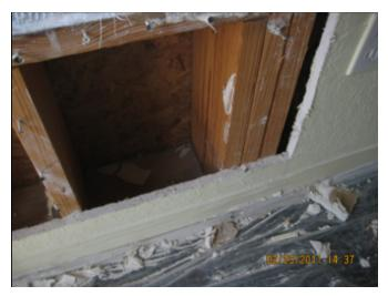
Figure 3 - Destructive Testing performed on interior face of wall
