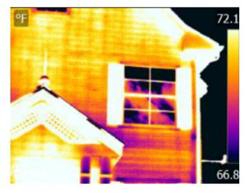
Figure 2 - Thermal anomalies at bottom left corner of window
