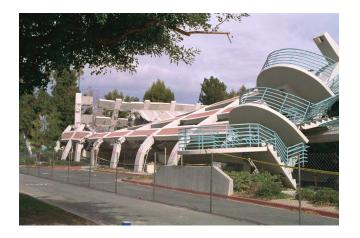
**Photo 4** - Structural collapse of a five-year-old parking garage in Northridge, California; 1994. (Credit: <u>USGS</u> <u>archive</u>)
