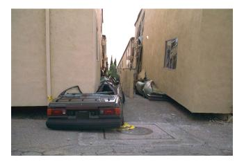
**Photo 2** - Soft story collapse resulting in crushed vehicles, (Credit: <u>USGS archive</u>)
