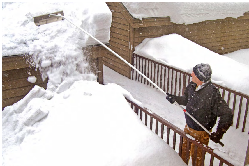
Figure 3 - Example of a roof rake being used to remove snow accumulation.
