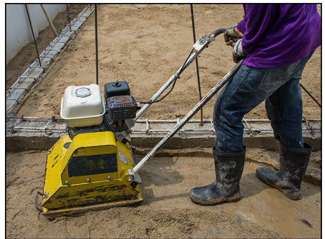
Figure 1 - Plate compactor in use on residential site
